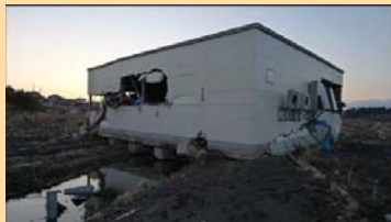
Building was carried 500m away by flood from its original site
